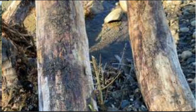
Figure 10. Close-up of willow and cottonwood cuttings placed within bank treatment after backfilling with channel sediment and trimming.
