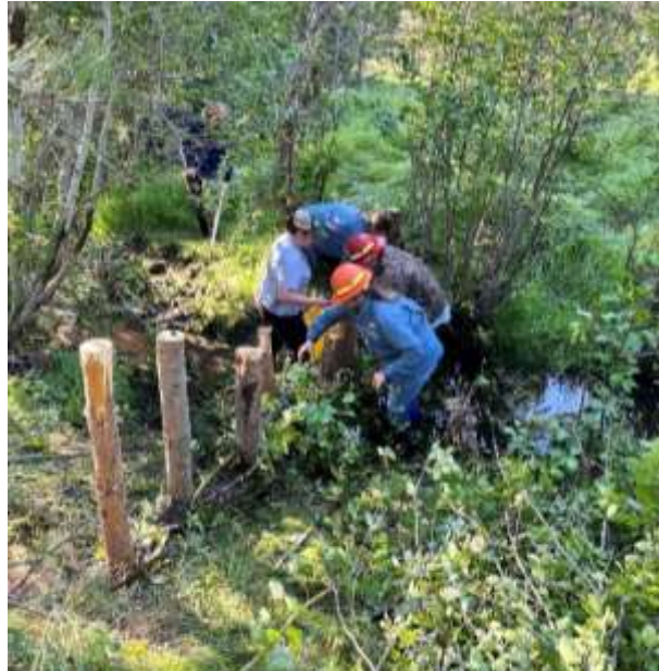
Figure 3. Youth crew constructing a BDA along Camp Creek, 2023.
