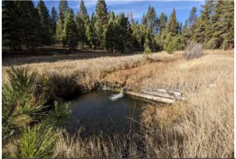
Figure 6. Camp Creek log weir fish passage barrier.
