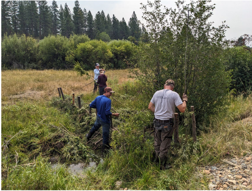
Figure 10: 2024 Beaver Dam BBQ participants construct BDA.
