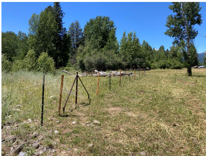
Figure 14. Riparian Buffer fencing installed along Pine Creek.
