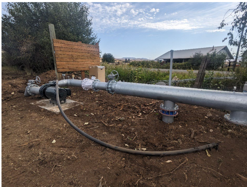
Figure 13: Completed pump station.
