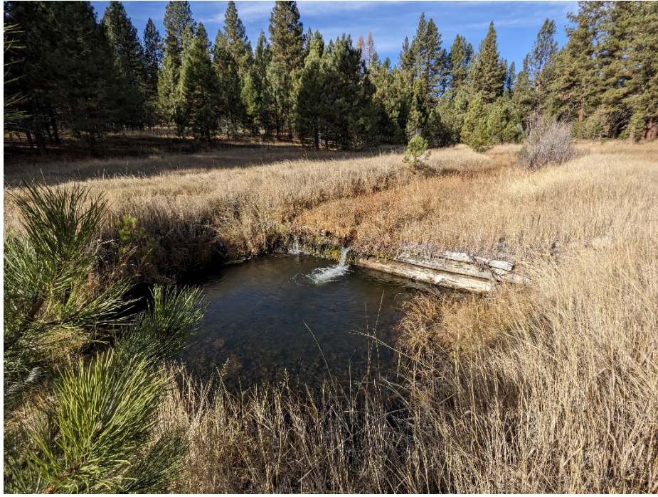
Figure 7: Log weir limits fish passage on Camp Creek.
