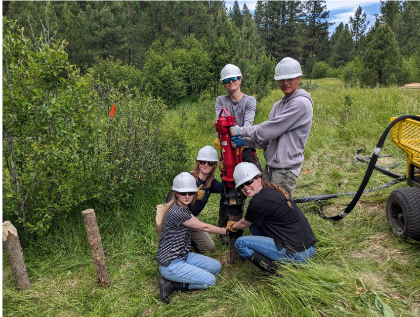
Figure 9: BRC 2024 summer interns pose with the post-driver.
