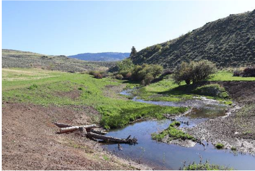
Figure 11. Cusick Creek showing bank pull-back, floodplain grading and wood structures.
